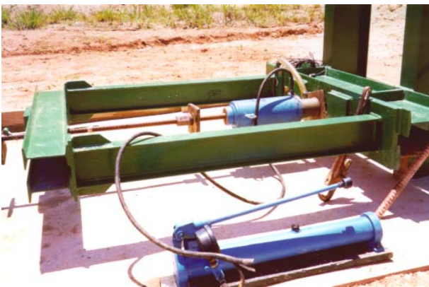
Figure 11. Reaction Structure and Hydraulic Piston
