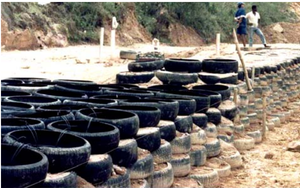
(c) Intermediate stage, section of cut tires tied with wire
