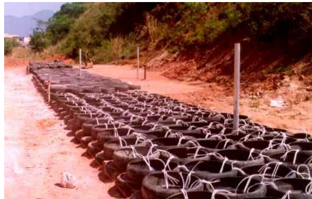
(b) Initial stage, section of cut tires tied with wire
