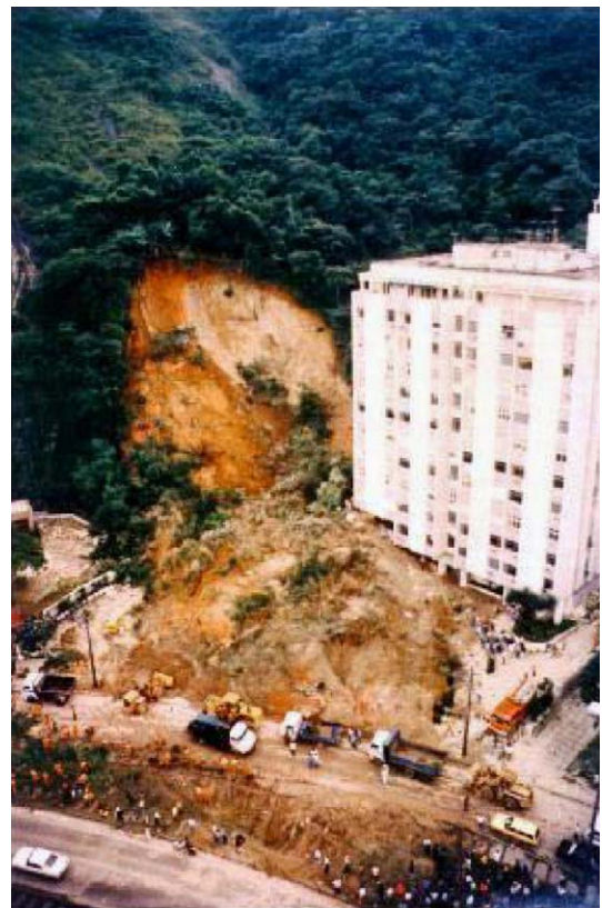
Fig. 2. Day after photo of Lagoa landslide.
