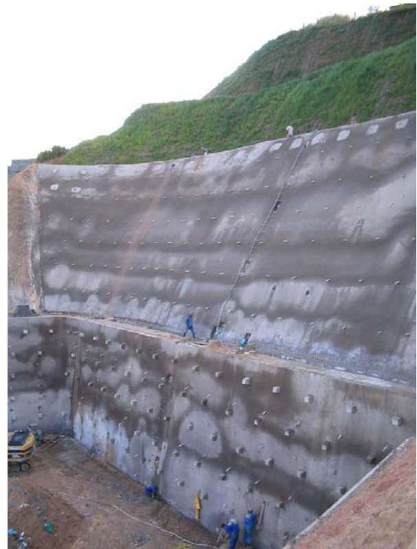
Figure 7 – Last stages of 40m high nailed excavation.
