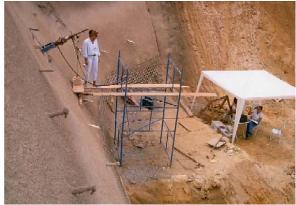
Figure 3 - Nail pullout testing on a platform during excavation.
