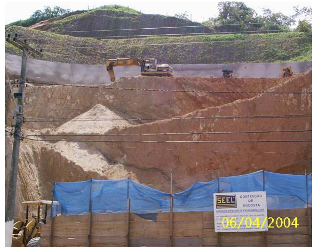
Figure 6 – First stages of nailed excavation.
