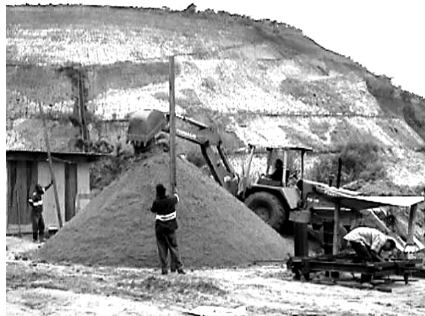
Figure 1. Field pullout test view.
